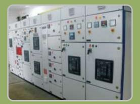
A distribution board is a component of an electricity supply system that divides an electrical power feed into subsidiary circuits, while providing a protective fuse or circuit breaker for each circuit in a common enclosure. Normally, a main switch, and in recent boards, one or more residual-current devices or residual current breakers with over current protection, are also incorporated.
